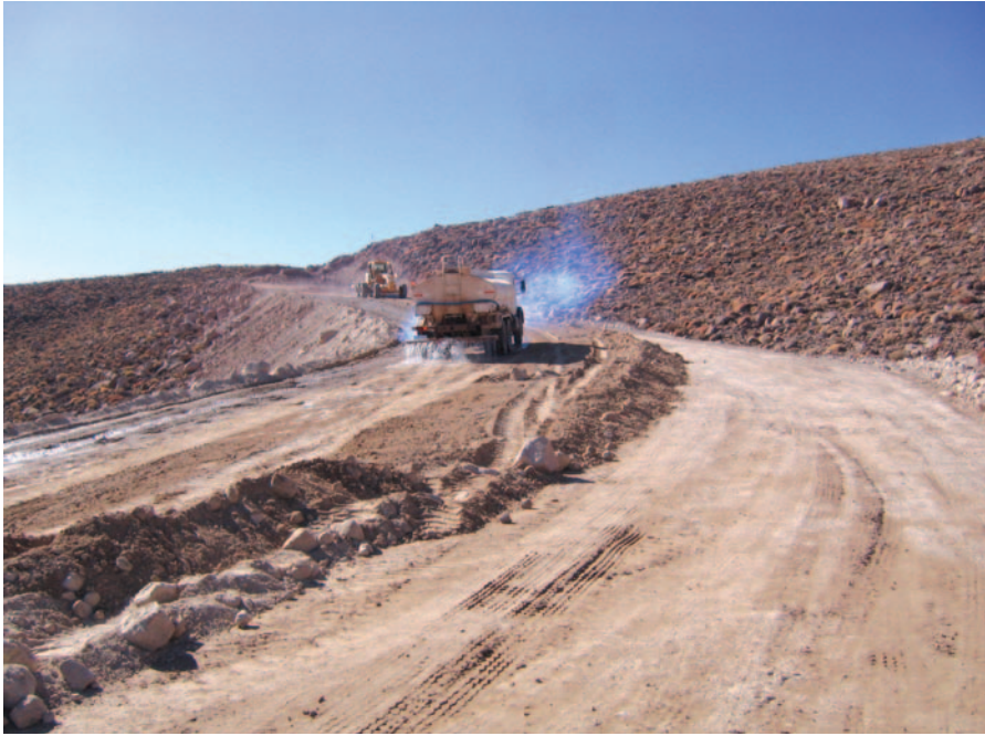
Figure 4: Construction of the 12-m wide road connecting the OSF to Llano de Chajnantor, the telescope site at 5000 m.
