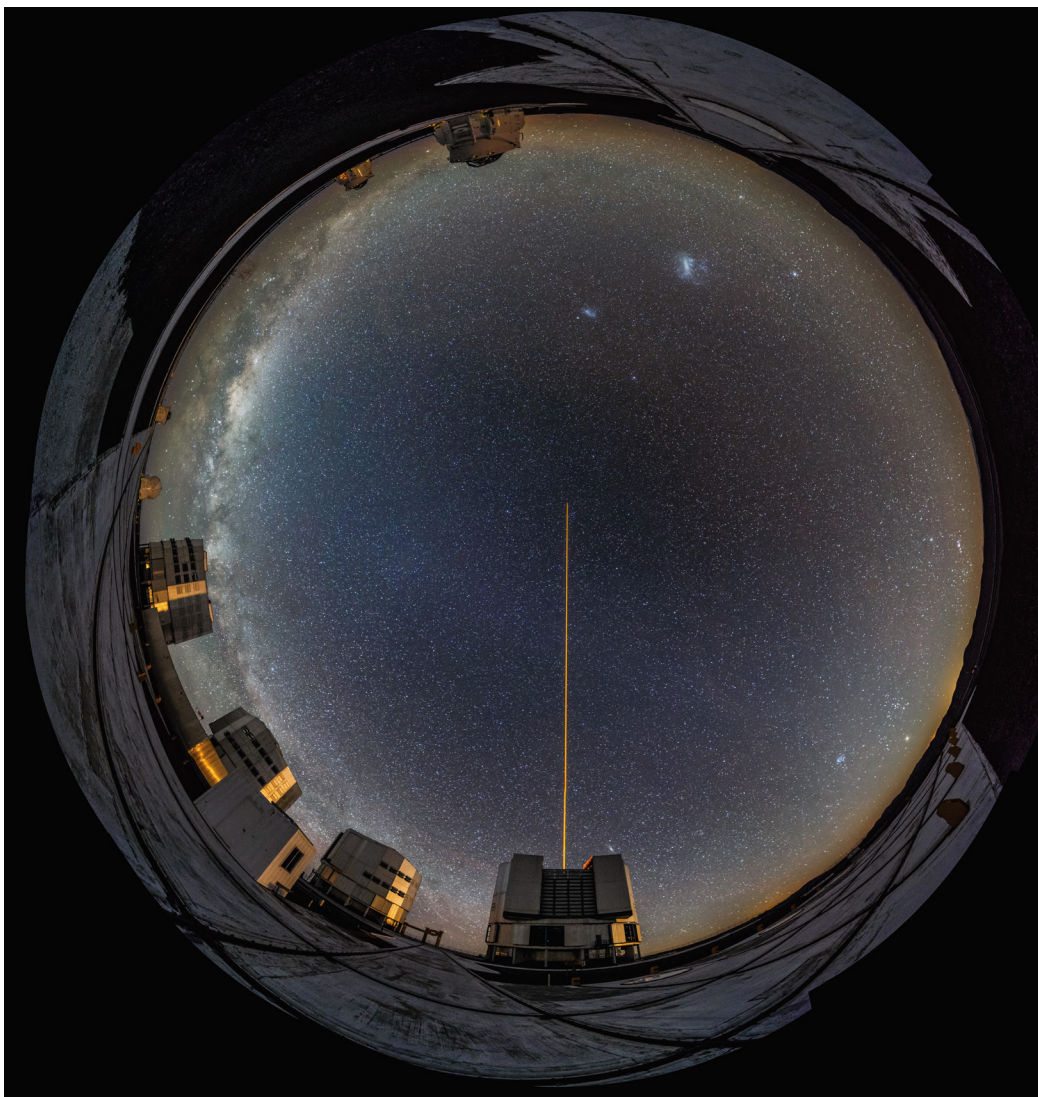
A fish-eye lens view of the Paranal Observatory, showing the four Unit Telescopes (UTs) and four Auxiliary Telescopes. The laser guide star emerges from the dome of UT4 (Yepun). The Large and Small Magellanic Clouds can be seen at the top of the image and the Galactic Plane near the horizon.
