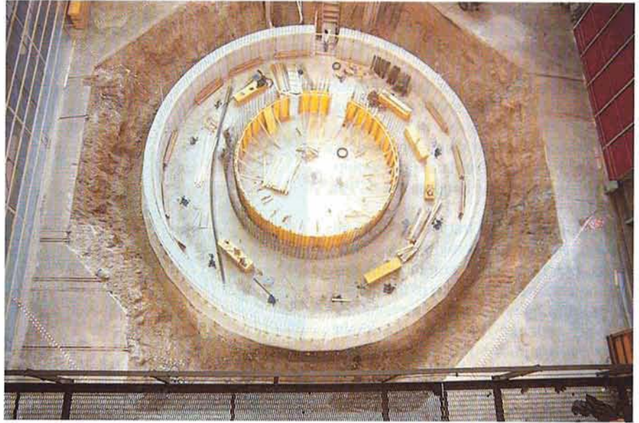
Figure 4: The telescope foundations in the test hall of Ansaldo in Milan.
