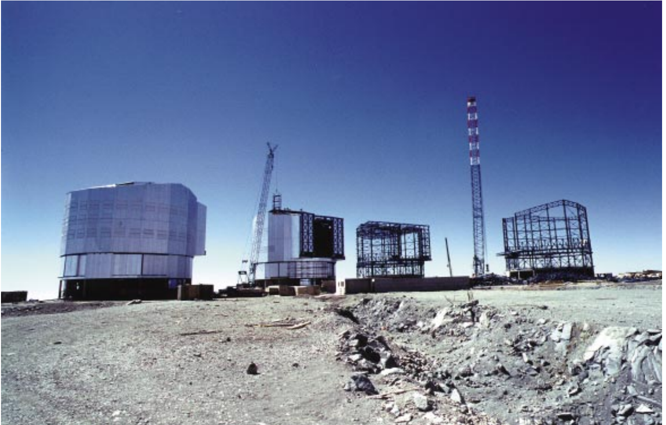
Figure 1 was obtained mid-October 1996 and shows the four enclosures at different stages of integration. No. 1 is complete, no. 2 is in the final stages of the implementation of the aluminium cladding, no. 3 is ready for enclosure cladding and no. 4 is in the final stages of steel erection which was completed the following day with the positioning of the roof using the 350-ton crane situated next to the dome.
