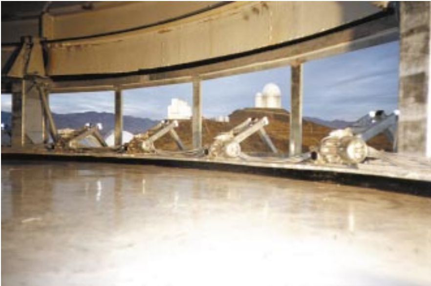
Figure 1: View of the open ports from the inside of the dome.
