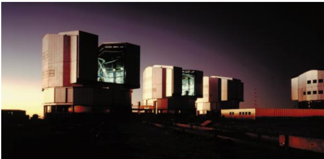
In this evening view, obtained about half an hour after sunset, the UT1 telescope structure is seen through the dome slit. The assembly of UT2 is well on its way in the next dome, and the first parts of UT3 are in place in the third.
